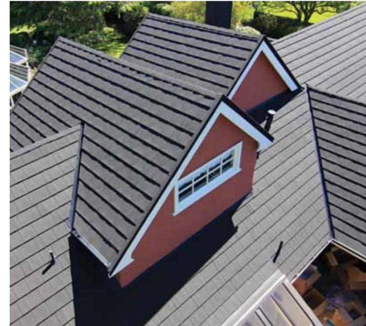
first being, that the replacement product had to compliment the original style of the house, and the low profile of the existing concrete roof tile. The Metrotile Shingle profile is unique in the New Zealand market, and it is the lowest profile pressed metal tile available. The
