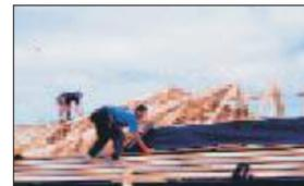
If the underlay is being placed over the plywood it is recommended that a hammer stapler be used to secure the paper before the tiles are laid.
